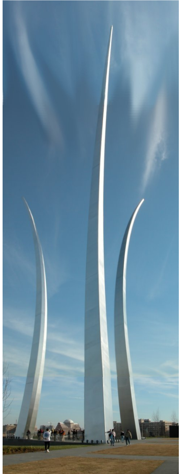
Recently completed Air force Memorial at Arlington, VA.
